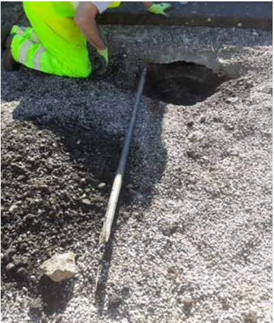
Photo 3. Pinch Bar positioned at the edge of foundation
