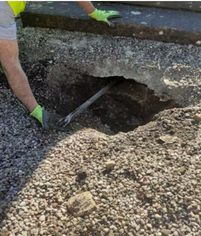
Photo 4. Pinch Bar positioned 1.10m into void space under foundation
