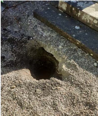
Photo 4. Pinch Bar positioned 1.10m into void space under foundation
