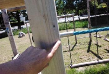
Finding: A number of fixing(s) have worked loose on the rope net
