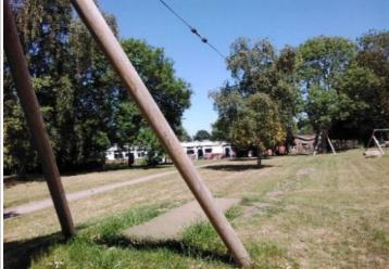
**Finding:** The seat(s) and suspension were missing at the time of inspection and the inspector was unable to make a full compliance assessment
