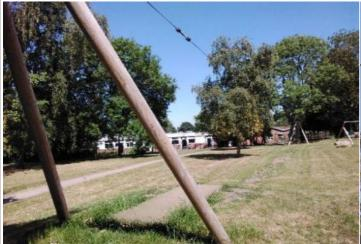
**Finding:** The seat and suspension are missing from the Cableway; ensure that the traveller is secured against use or removed to prevent misuse
