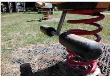
Finding: A number of fixing(s) have worked loose securing Action: Secure all loose fixings the foot rests
