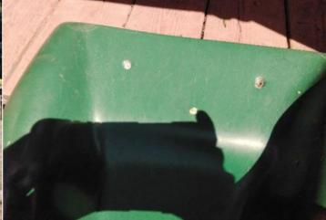
Finding: There is damage to the slide gel coat
