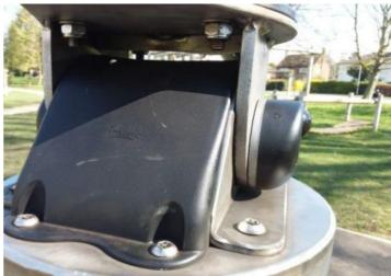
**Finding:** There are missing spaces on the mount plate or they have been over tightened which is causing them to wear
