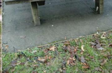
Finding: There are trip hazards at the edges of the surface Action: Reinstate surrounding surface levels to remove the trip points
