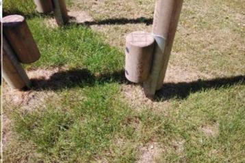
**Finding:** A number of fixing(s) have worked loose in the stilts posts
