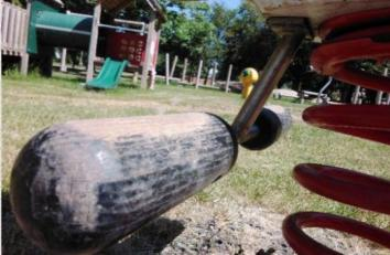
**Finding:** A number of fixing(s) have worked loose on the foot rests
